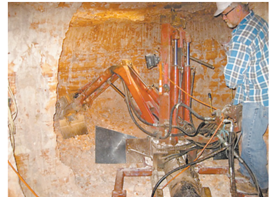
UNDERGROUND WITH HYDRAULIC ROTARY HEAD DIGGER; LARGE BLACK PIPE SUCTIONS UP DIRT FOR PROCESSING. COURTESY JOHN TERNUS, OPAL GUY.
